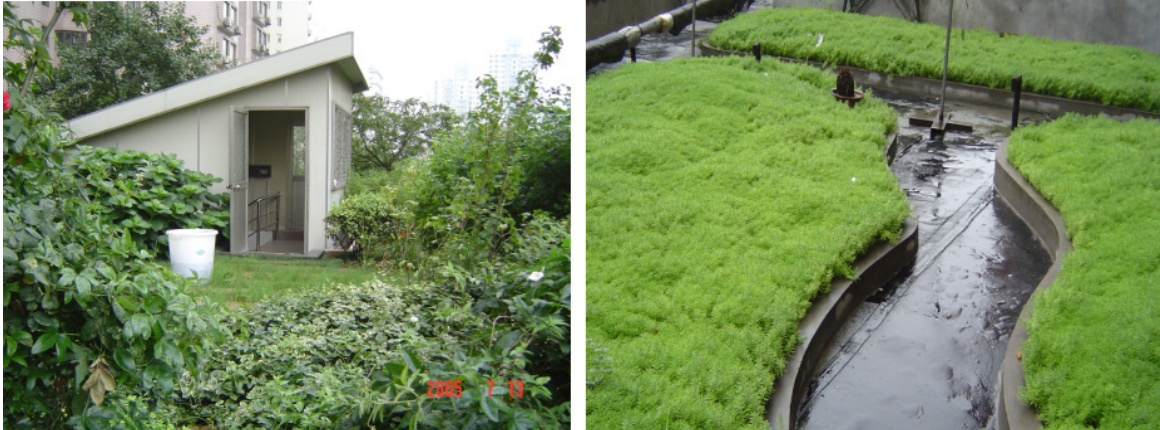
Plants growing on roofs(in Shanghai Jingan greening bureau )
